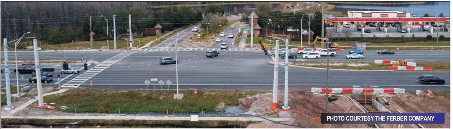
Underground piping plus light and power poles are installed along 54 before Ballantrae’s entrance is widened by two lanes in coming months.
