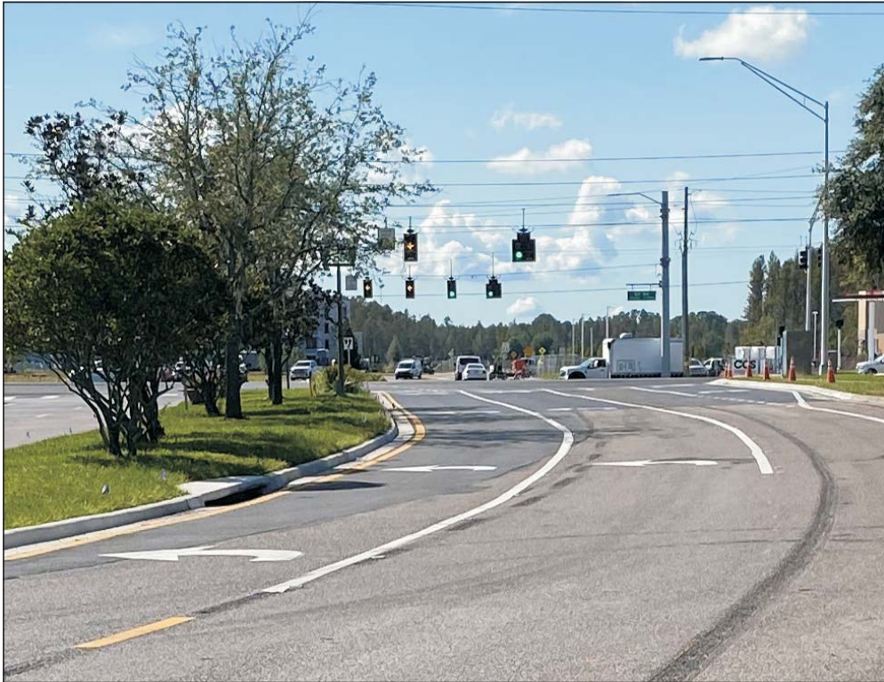
Ferber has finished paving and striping Ballantrae Blvd.'s four southbound lanes.
